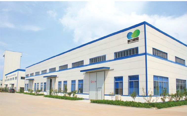
生产加工车间外景 Production And Processing Workshop Exterior
