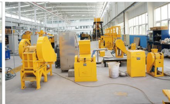
矿物破碎加工区 Crushing Area
